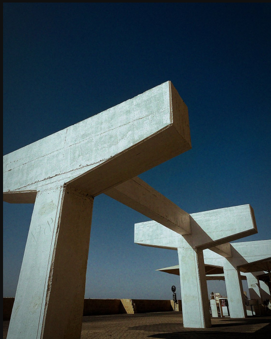
Concrete t forms. Citus Camera, G200 100% · grain 40/50 · clarity +16, structure +35 · highlights -100 · vignette 36. 15 Sep 2026. Photograph by Leon Yakobov.
